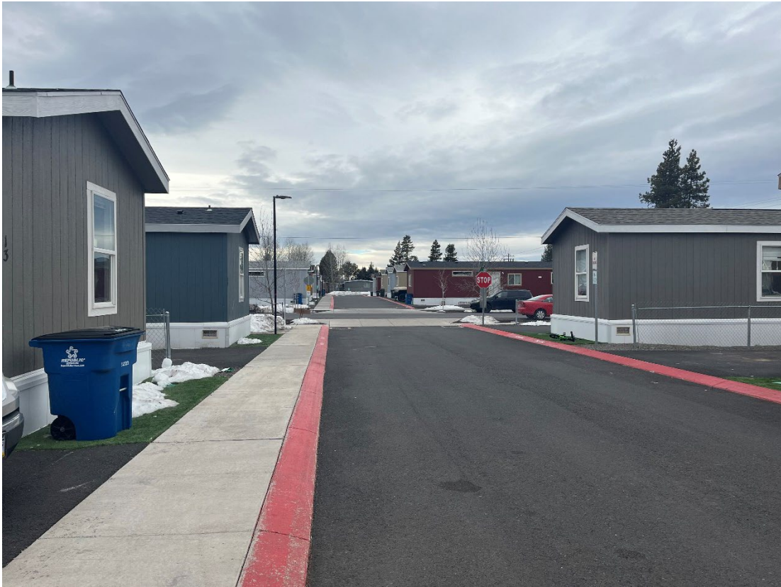
Figure 5: View of the sidewalk within the park looking west.
