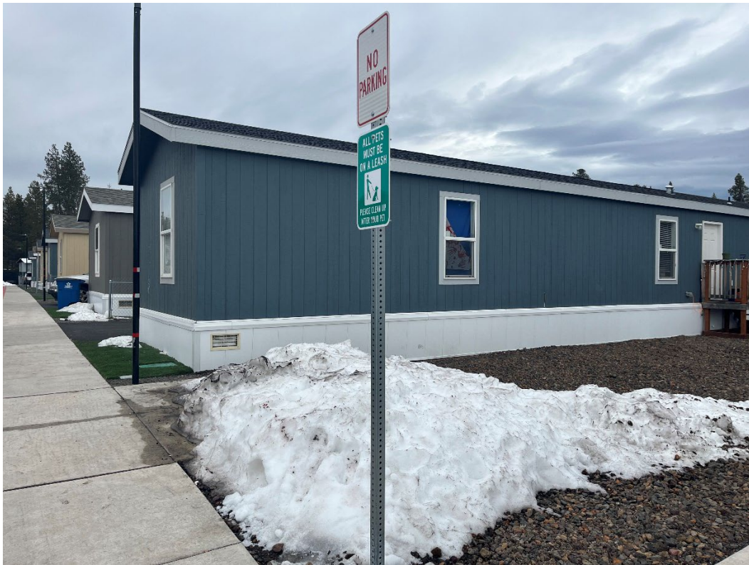
Figure 3: One of the dwellings located at the entrance on Preble Way.
