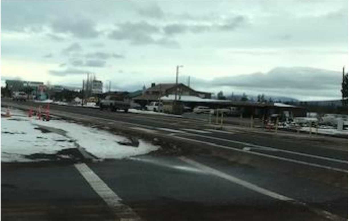
Figure 13. US 97/Finley Butte Road intersection facing south showing the newly installed raised pedestrian refuge island and sidewalks.
