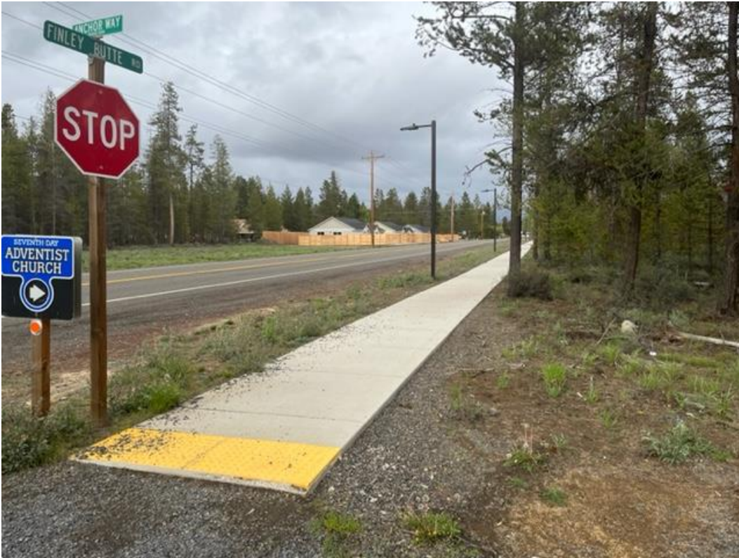
Figure 9. View from Anchor Way facing east along Finley Butte Road.
