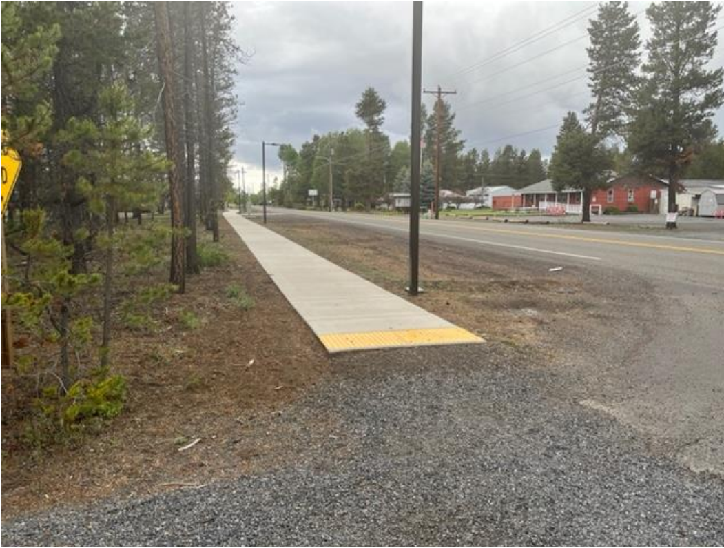
Figure 10. View west along Finley Butte Road at Anchor Way.
