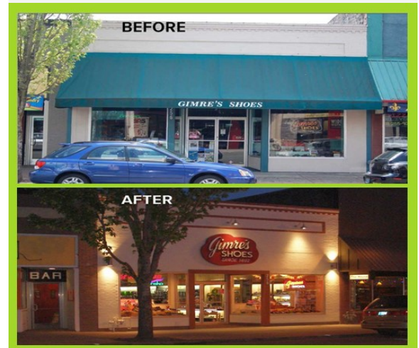
Façade improvement to existing building.
