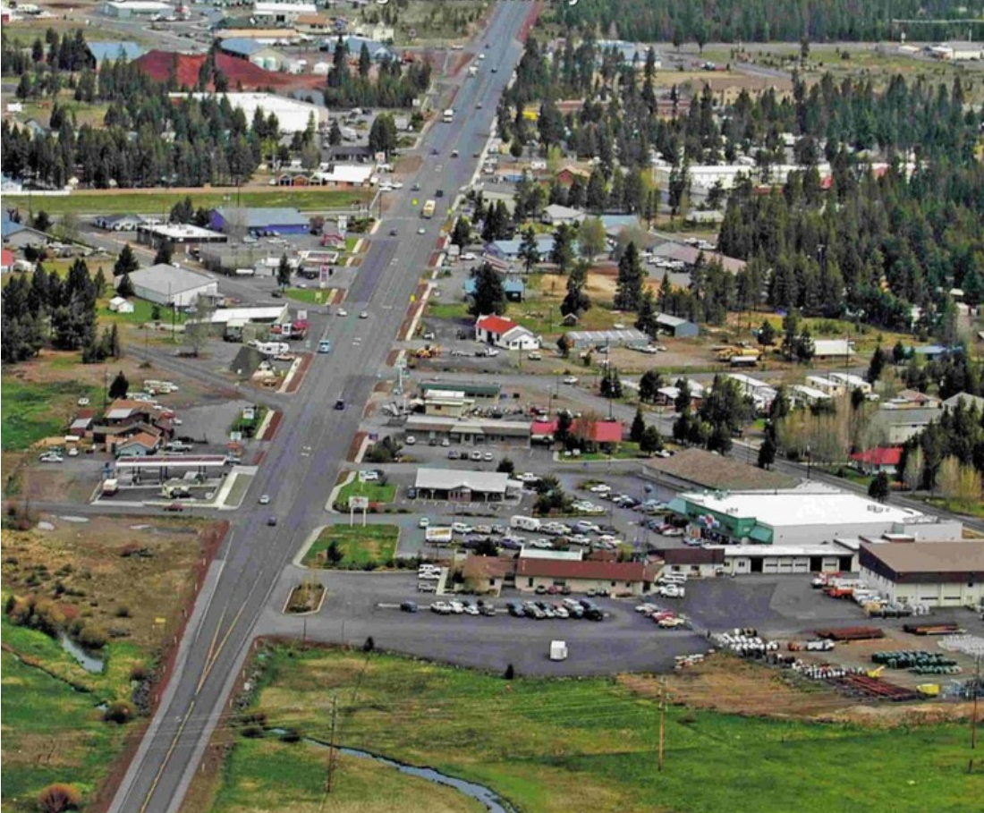
Aerial view of the Highway 97 La Pine commercial corridor
