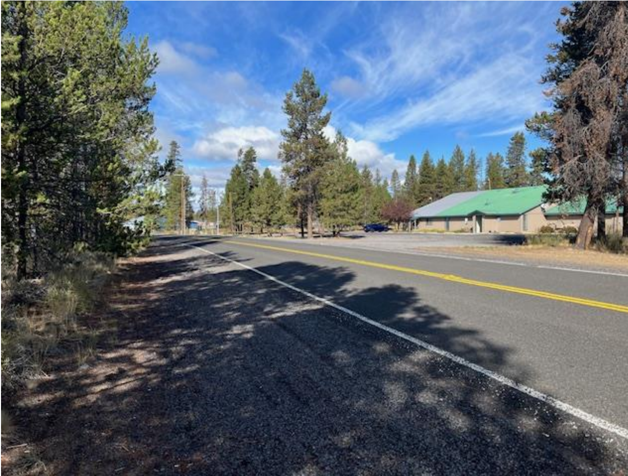
Figure 12. View along Rosland Road facing west. Photo date: September 2023.
