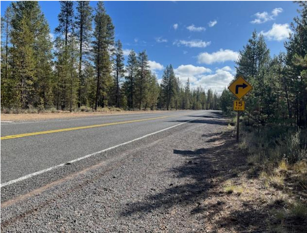
Figure 11. View along Rosland Road facing east. Photo date: September 2023.
