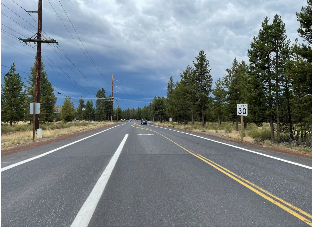
Photo 1: Looking south from 400 feet north of Memorial Lane.
