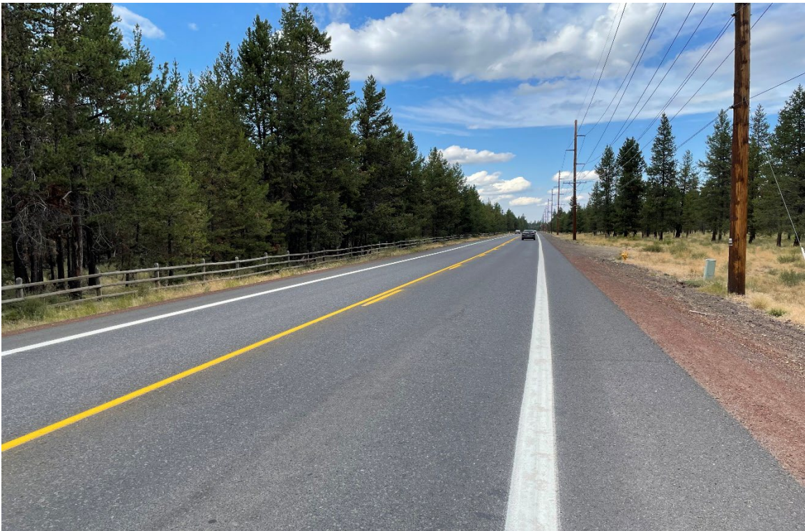
Photo 8: Looking north from 350 feet north of Findley Drive.
