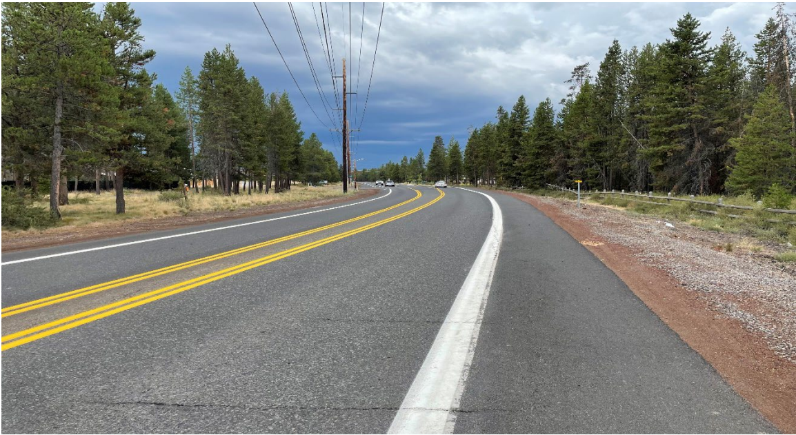
Photo 3: Looking south from 350 feet south of Pengra Road.
