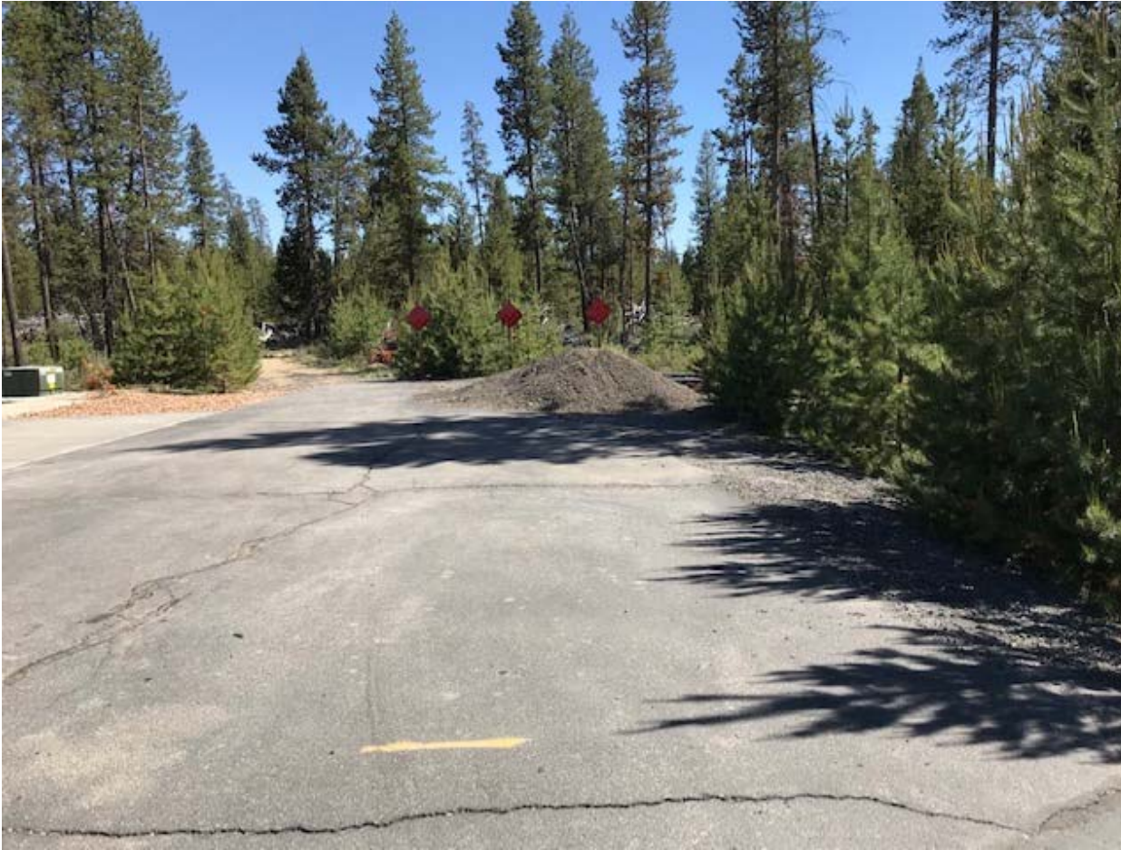
Figure 13. View of the southern terminus of Wheeler Road.
