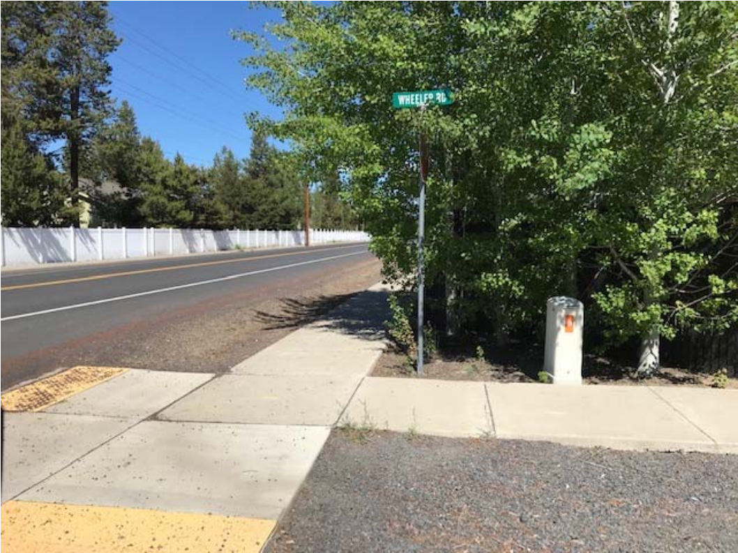
Figure 10. View east along Finley Butte Road at Wheeler Road. It is recommended that the adjacent tree be trimmed to provide clear visibility to the stop sign and along the sidewalk.
