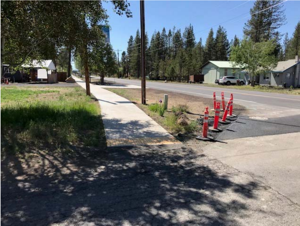
Figure 8. View west along Finley Butte Road at Walling Lane.
