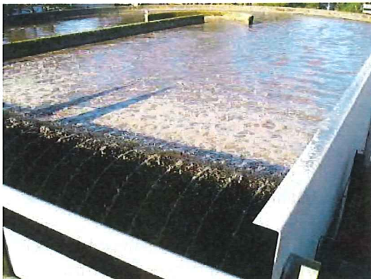
Seaside Wastewater oxidation ditch
